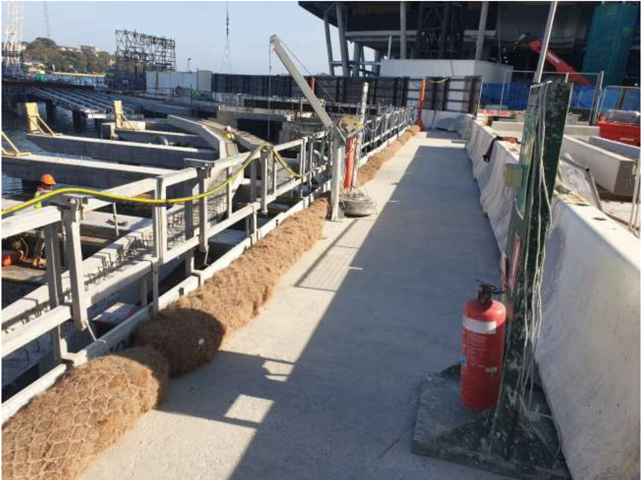
Photo 2: Coir logs on water's edge
