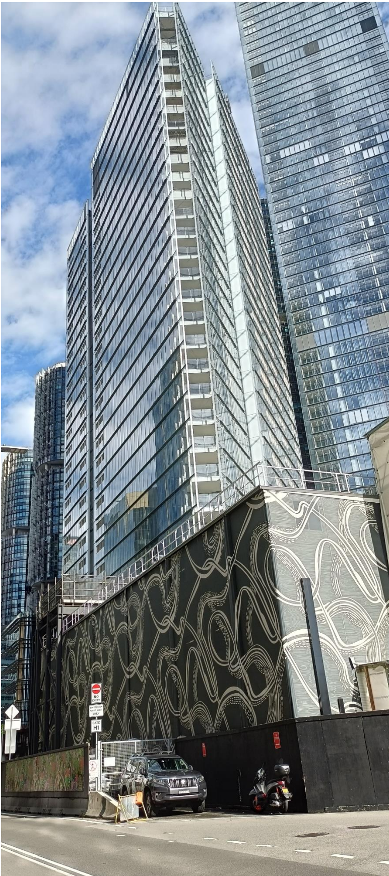
Photograph B.1 External building from Hickson Road
