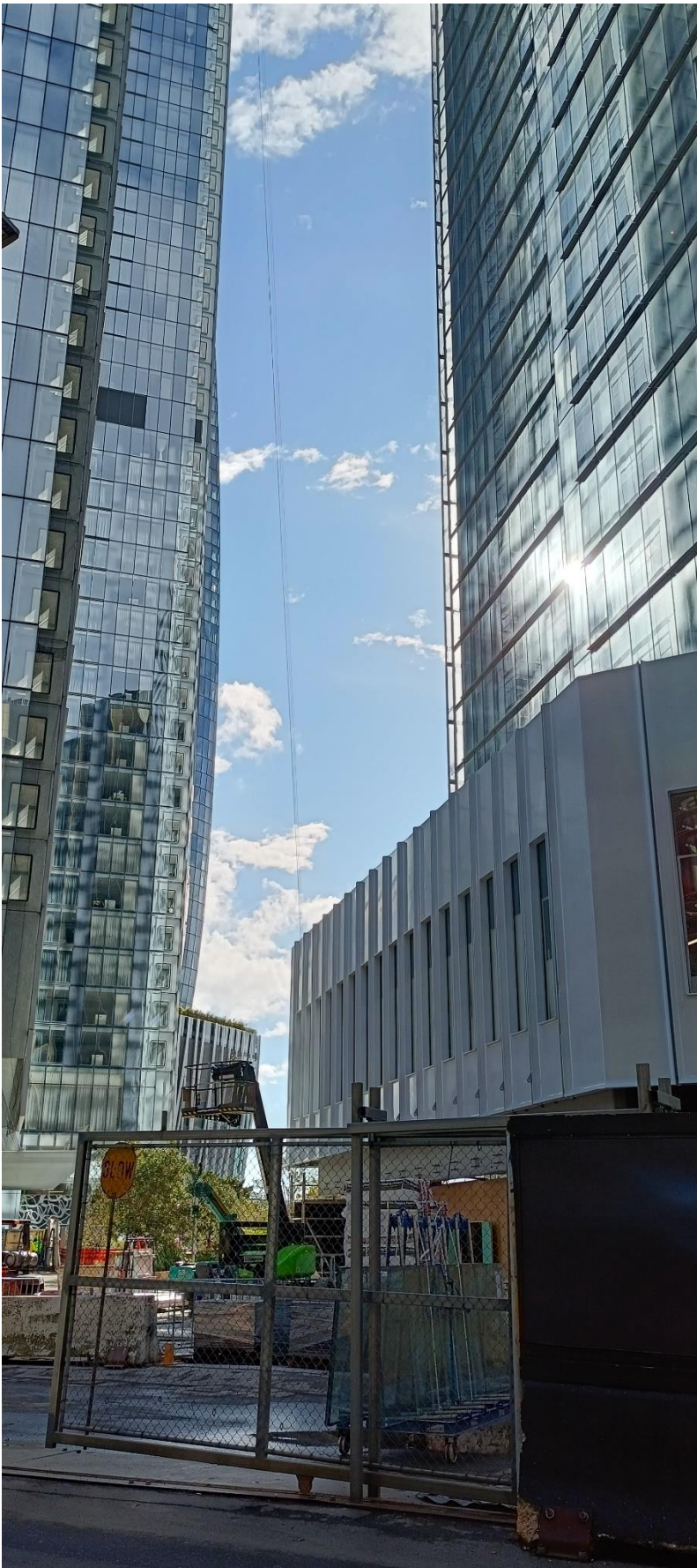
Photograph B.6 View from Watermans Quay showing Podium level and hording removed to Hickson Park
