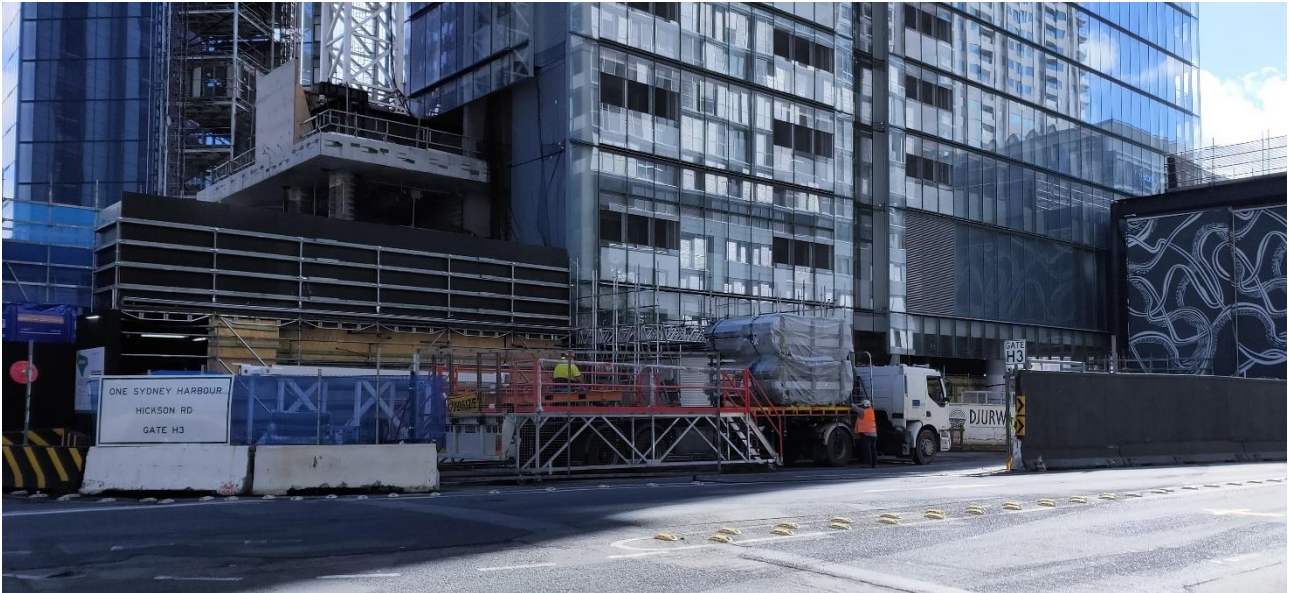
Photograph B.3 Gate H3 layout and signage off Hickson Road
