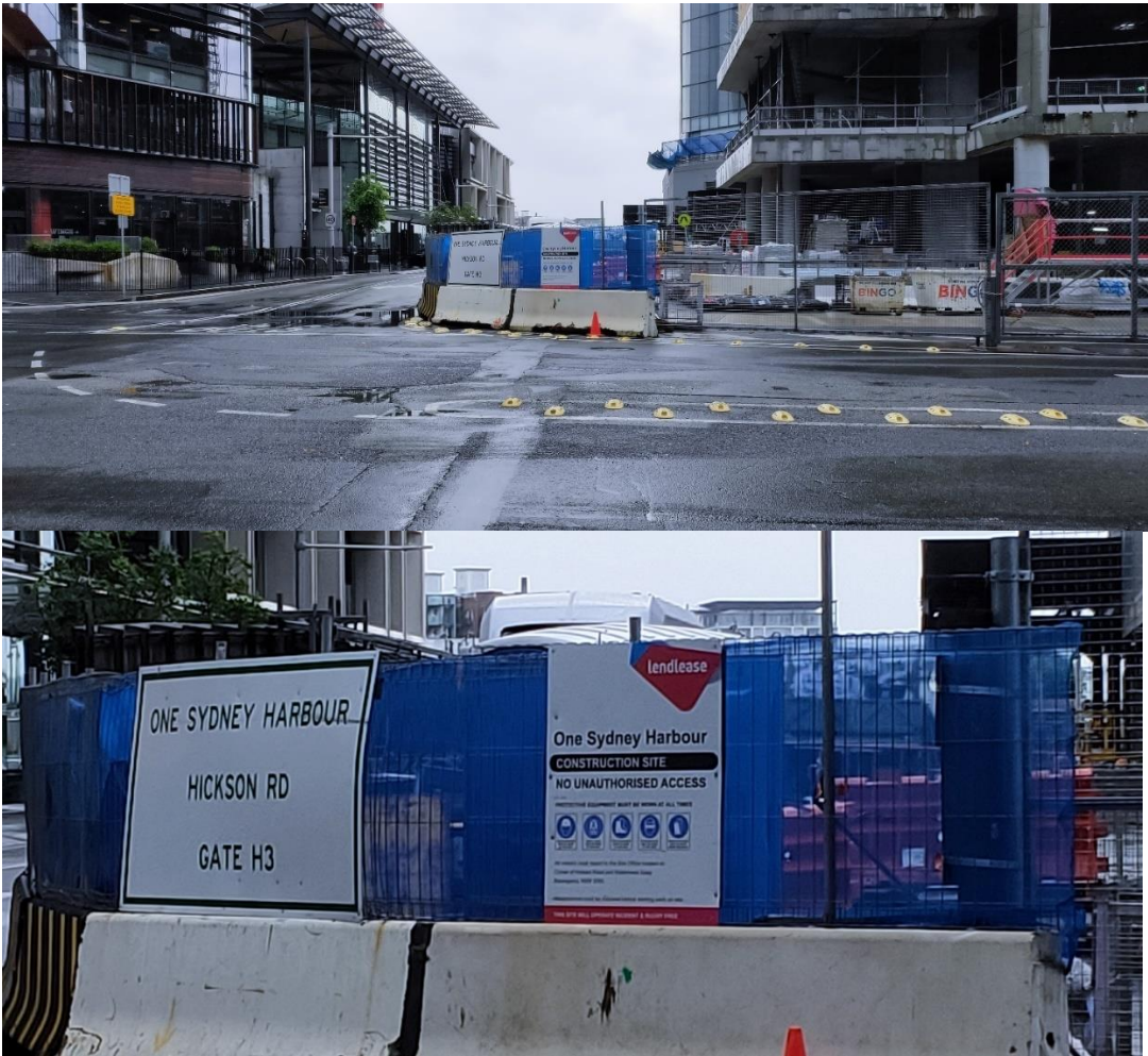
Photograph 5: Hickson Road looking West with project signage in place.
