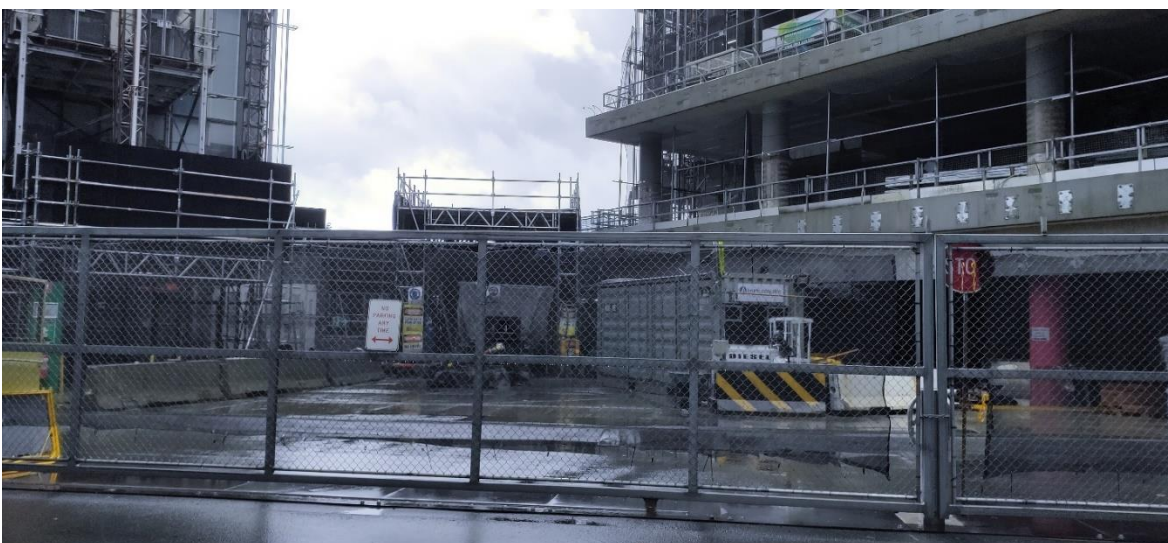
Photograph 3: Waterman Quay Rd looking North showing sound proofing on concrete pumps.
