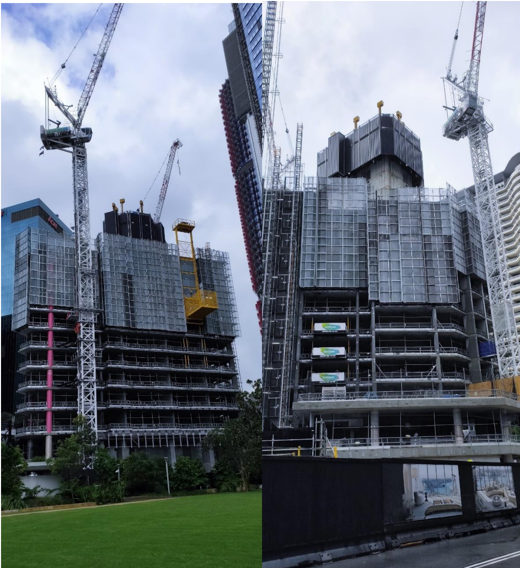
Photograph 1: External building from Hickson Park
