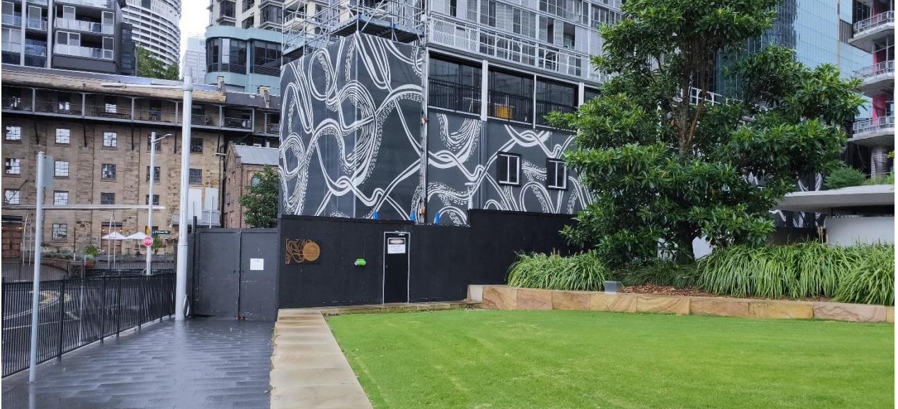
Photograph 6: External building and hoardings around Hickson Park and Hickson Road
