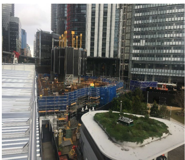
Roof top view into the site.
