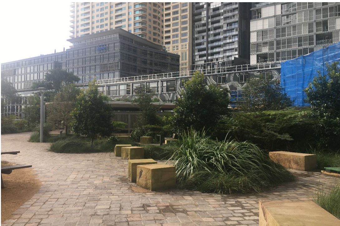
External view - Hickson Park Public toilets looking north
