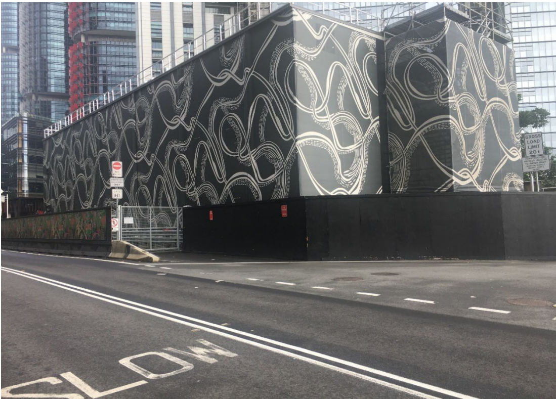
External view - Hickson Rd looking south
