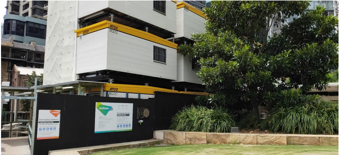
Photograph B.5 Hickson Park site entry with project signage in place
