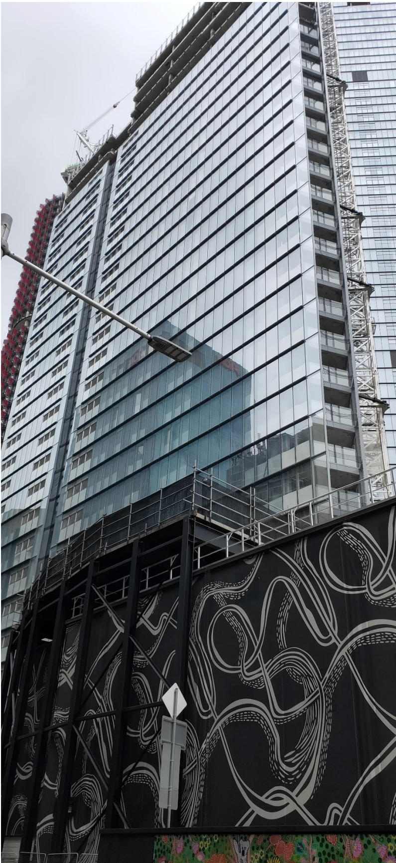
Photograph B.1 External building from Hickson Road
